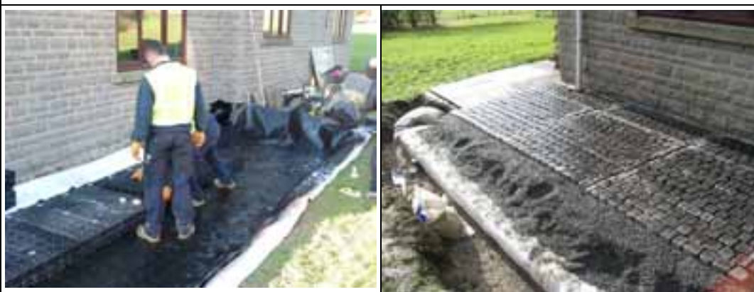
Installation of a rainwater harvester system below a permeable concrete block surface
